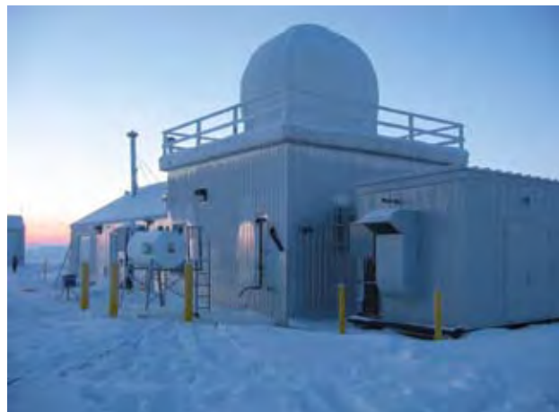
A Comprehensive Test Ban Treaty Organisation Radionuclide monitoring station
